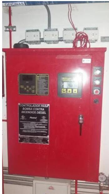
Fig. 11 Tablero de Control ECI Mall
