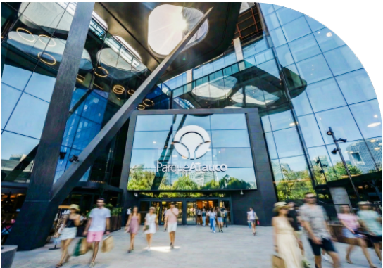
Parque Arauco Kennedy Expansion - Cerro Colorado Phase
